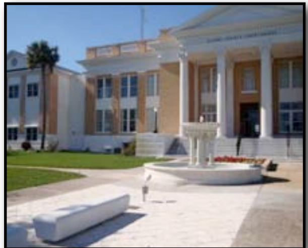
Glades County Courthouse after external renovations: Fountain was added to the walkway, along with benches, a flower bed at the base of the stairs and lighting. Also, sod was added to create 3 lawns separated by converging sidewalks at the fountain.
