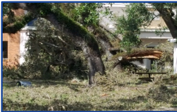
Outside Hendry County Courthouse after Irma
