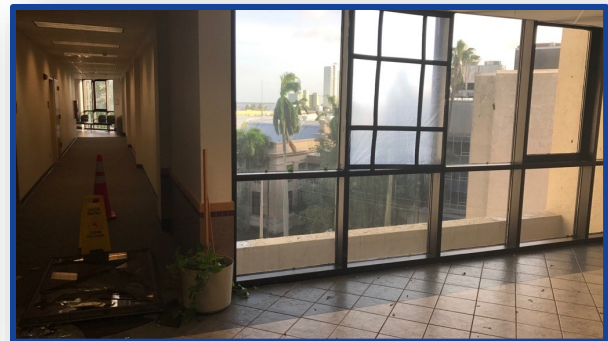
Damage on 5th Floor of Lee County Justice Center after Irma
