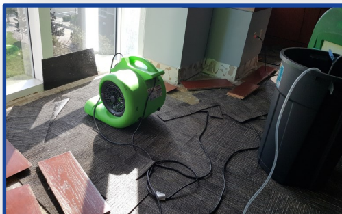
Damage in Charlotte County CR 3A after Irma
